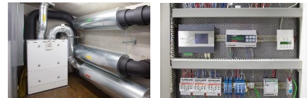
Construction of a residential house in Oberbayern (Germany)
