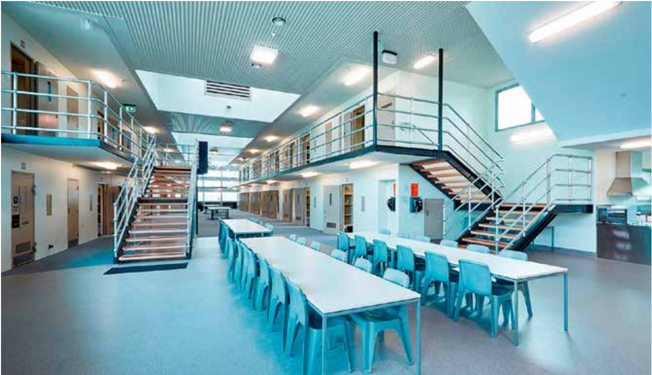
Adapted lighting conditions support detention management and energy efficiency.
