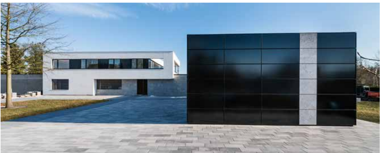
Bold architecture: Energy Plus house with KNX home automation.
