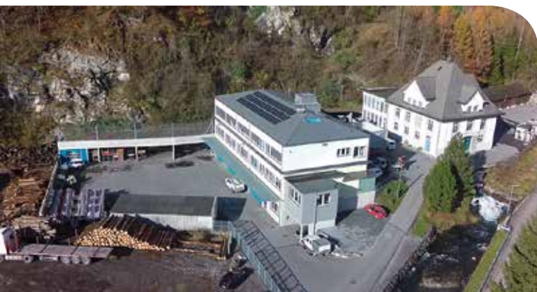
Compliance with energy efficiency classes: KNX integrates all trades in the office of the department networks which is located in the new work yard
