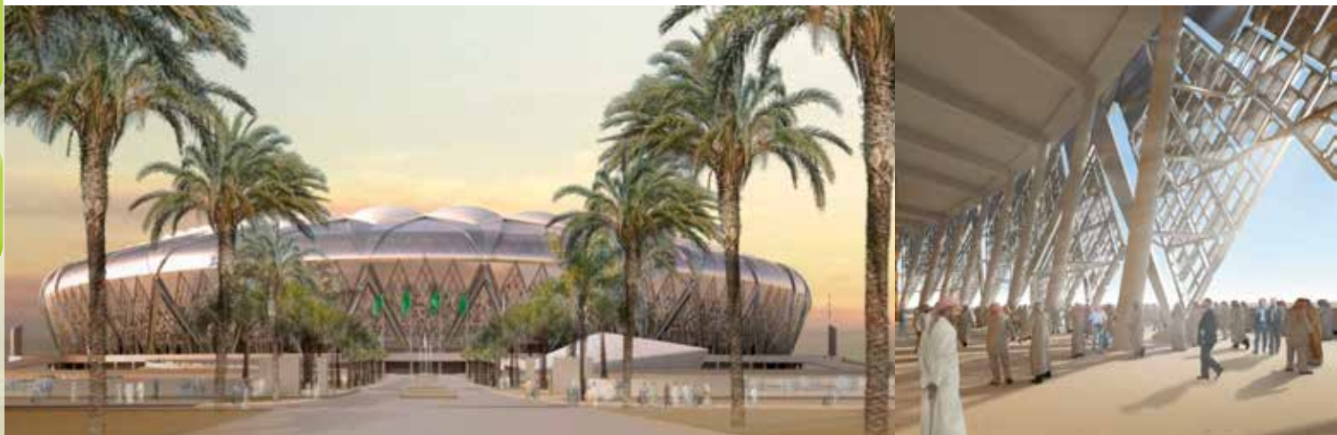
Jewel in the desert: KNX controls the lighting in the second largest stadium of Saudi Arabia.
