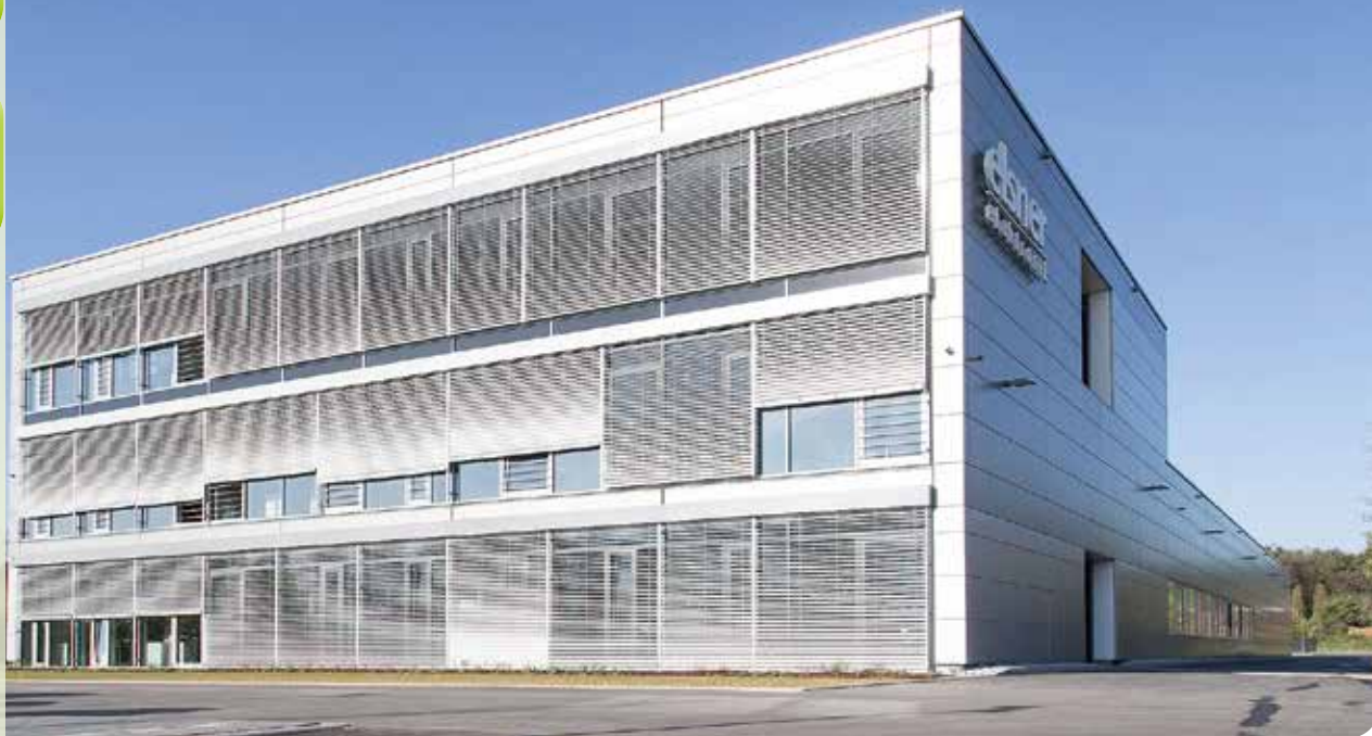
Individual control of the sun screens is released
