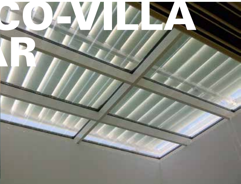
Automatic sun protection provides on hot days comfortable shade in the atrium
