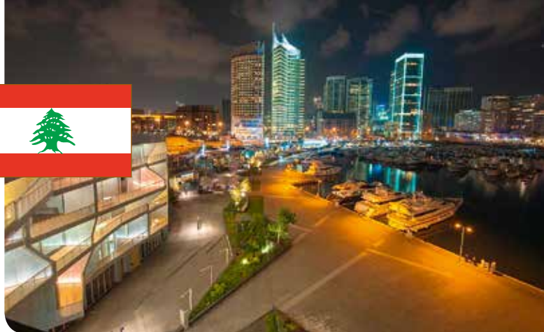
Le Yacht Club Beirut, a KNX installation of over 900 KNX devices for controlling lighting, shutters and HVAC.
