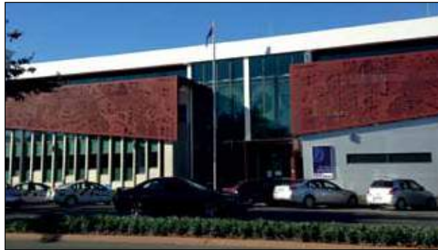
The new Rotorua Police Station incorporates KNX technology.
