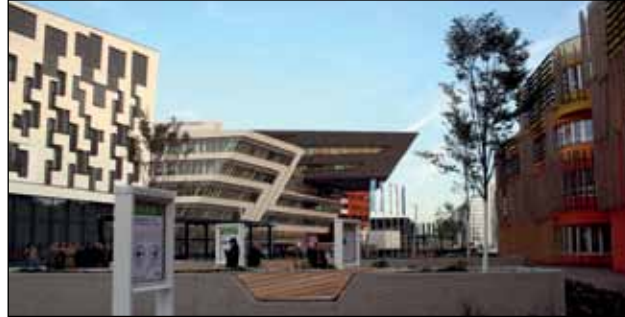
Different architectural styles on the outside, but just one KNX-based concept on the inside – the new campus of Vienna University of Economics and Business.
