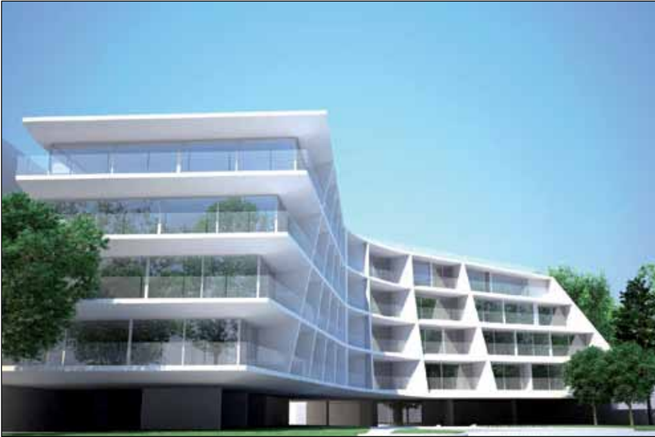
Every evening a perfectly tailored KNX-controlled lighting system brings out the best in the development's contemporary architecture.
