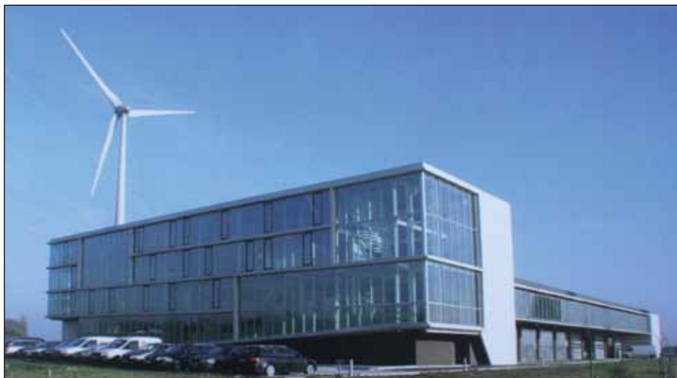
Behind the contemporary architecture, KNX provides energy efficient building automation.
