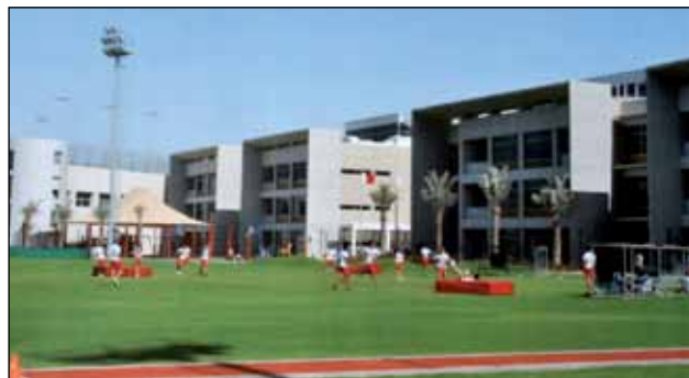
Pupils at the American School of Dubai. KNX is in charge when it comes to the building services – that ensures maximum energy efficiency.
