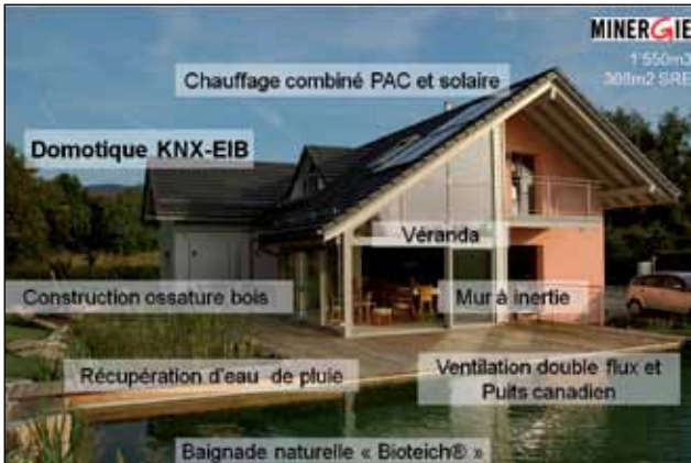
KNX based controls and analysis of energy consumption data have resulted in considerable energy savings at Villa Minergie.
