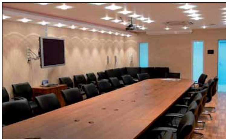
Intelligent building automation functions were demonstrated in the meeting room
