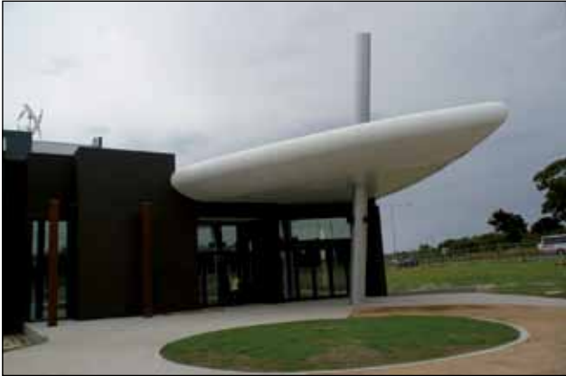
Environmental protection and sustainability are valued highly on the Surf Coast. The efficient building system technology with KNX meets this requirement
