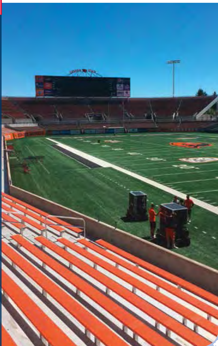
Reser Stadium upgrades to a KNX lighting system
