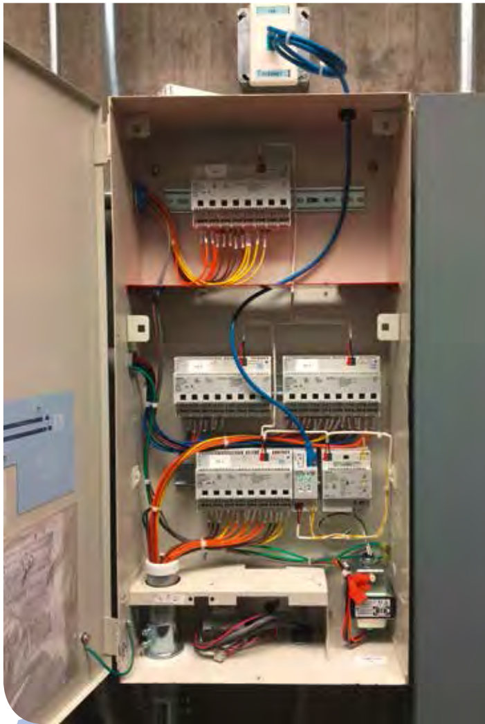
The GAMMA system features a distributed control architecture that lets the stadium easily manage all aspects of lighting.
