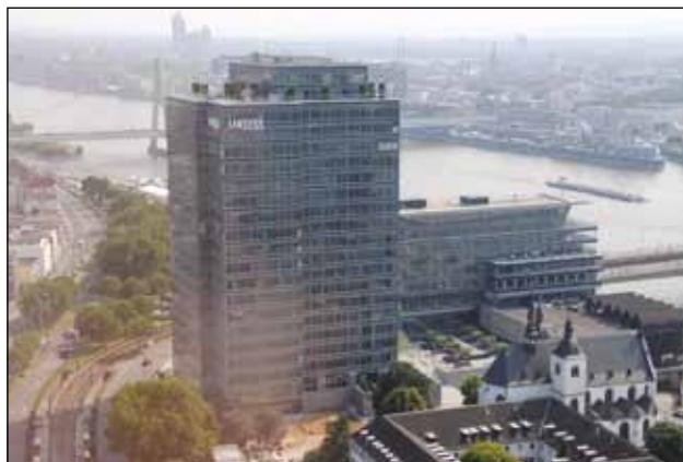
KNX automation helped improve the energy efficiency of the Lanxess Tower and the adjacent Rhein-etagen.
