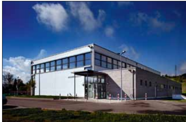
Heat from the sun provides welcome warmth in winter, but in summer, an automatic solar shading system keeps the building cool and protects sports hall users from glare
