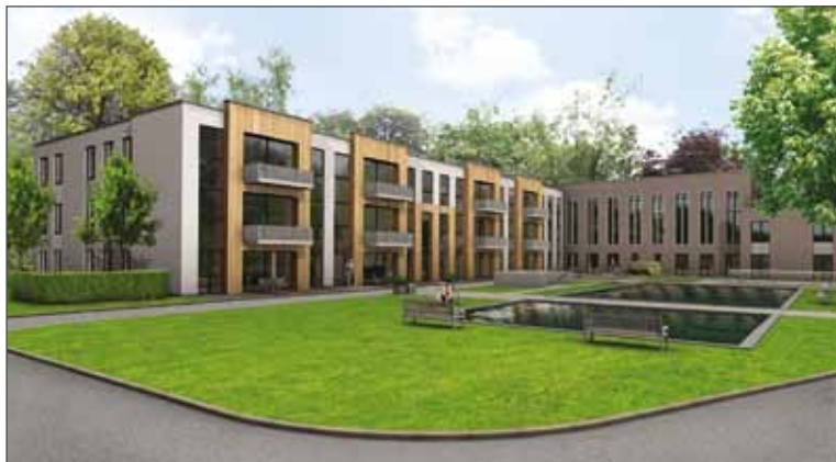
Independent living in green surroundings – KNX keeps energy costs under control
