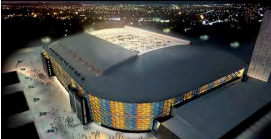
Friends Arena – the newest eye catcher in Stockholm is controlled by KNX.
