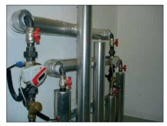
Figure 1. Heat meters with M-Bus interface and M-Bus-KNX-Gateway
