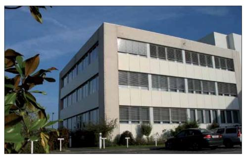
A sensor-controlled sun protection system reduces the cooling load
